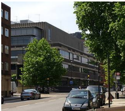
One of the three CCC centres. Note the array of Airwave antennae on the roof
